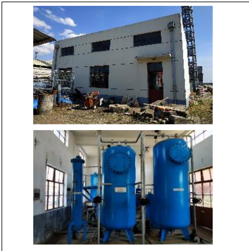
Figure 3.4-11 TJQ 5T/h Air Floating Water Purifier (Wastewater Treatment System)
